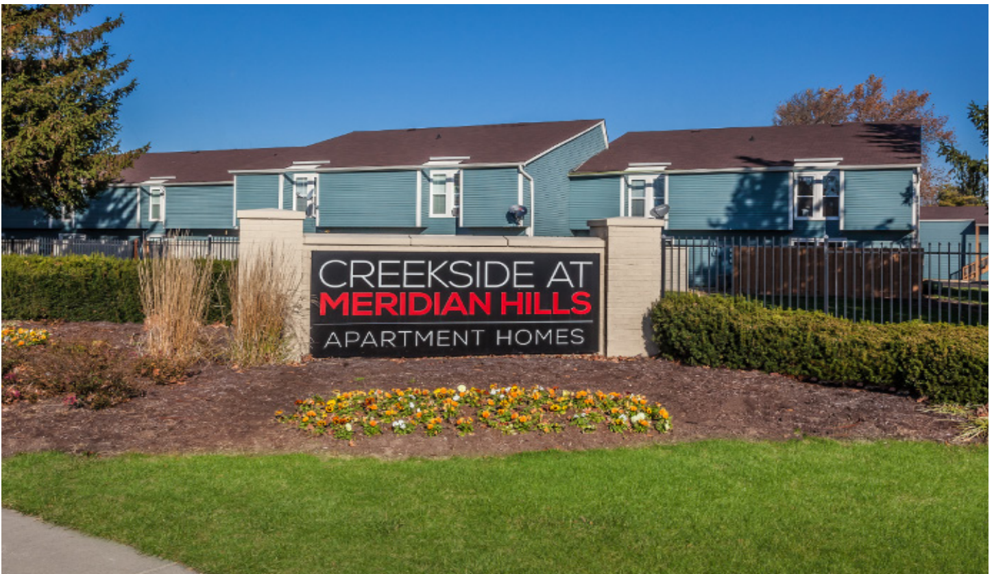
Creekside at Meridian Hill, Indianapolis, IN
