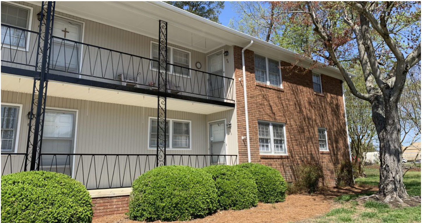
Briarcliff Apartments, Wilson, NC
